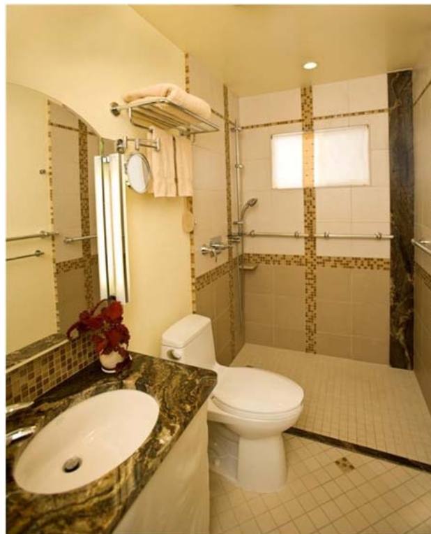
Regan's focus on accessible design can be seen in this bath's completely barrier-free shower design.
